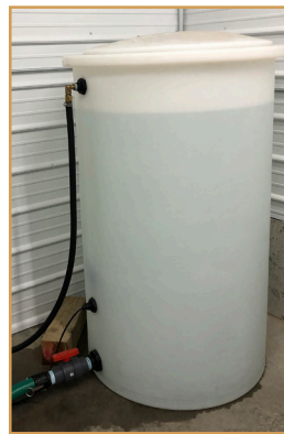
250-gallon holding tank, floats and supply plumbing
