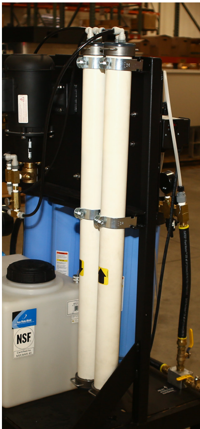
Reverse Osmosis Membranes
